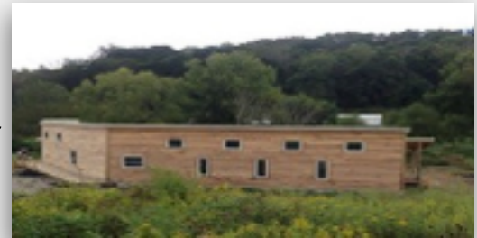
The Ups Center for Medicinal Plants under construction
